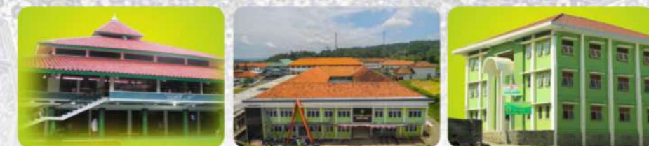
Masjid Annur SMK Wicaksana Gedung STAIA
